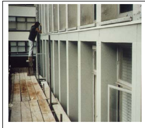
Figure 1b Cosmetic overcoat applied
