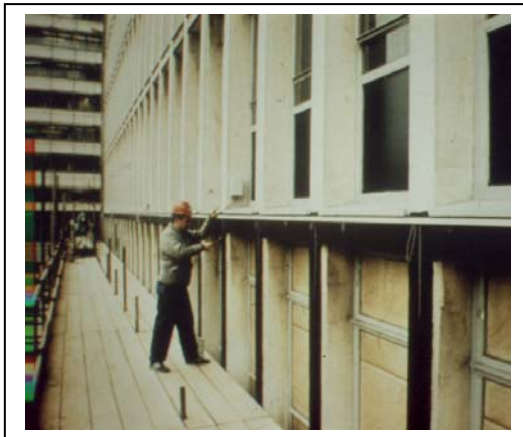
Figure 1a Conductive coating on front face
